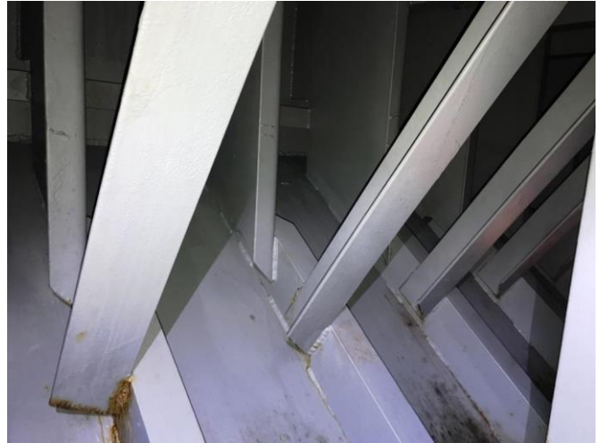
Photo # 16 – Bow rake trusses at the Headlog
