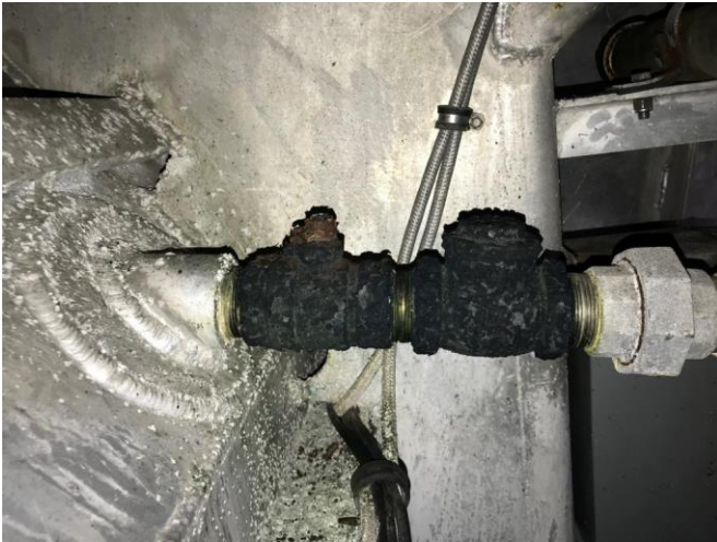
Photo # 57 – Comp. # 4 – Corrosion at overboard discharge
