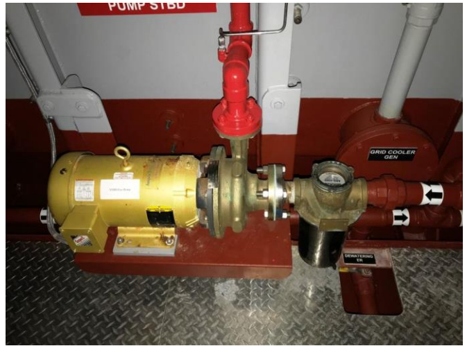
Photo # 30 – Main fire pump starboard side
