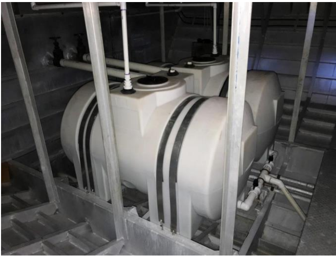
Photo # 37 – Comp. # 3 – Sewage holding tanks
