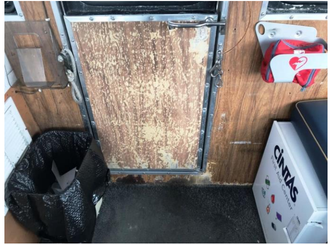
Photo # 24(a) – deterioration of joiner work at doorway
