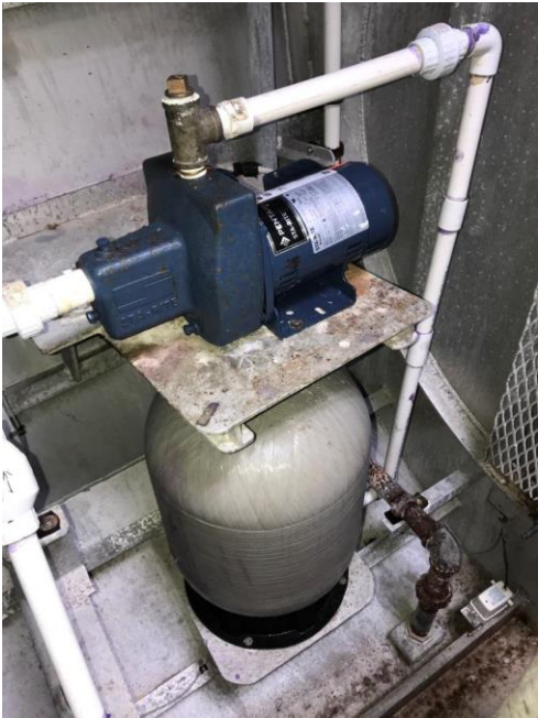
Photo # 45 – Comp. # 3 – 8.5-gallon fresh water pressure set
