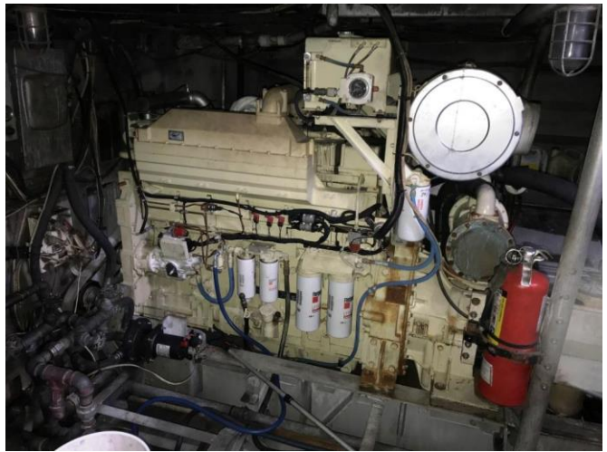
Photo # 32 – Comp. # 4 - Starboard main engine – 640 HP
