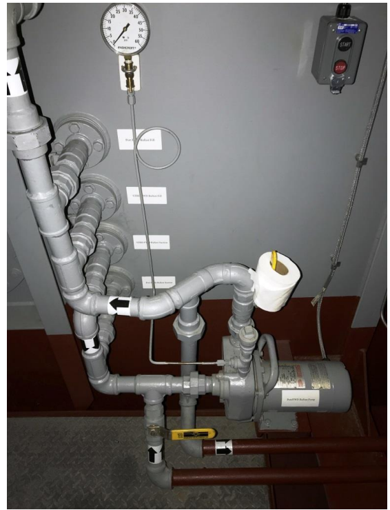
Photo # 34 – Ballast pump & Manifold
