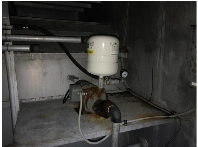
Photo # 56 – Comp. # 6P – Fresh water pressure set
