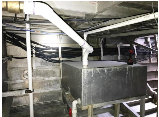
Photo # 30 – Compartment # 3 – looking to port showing portside sewage holding tank
