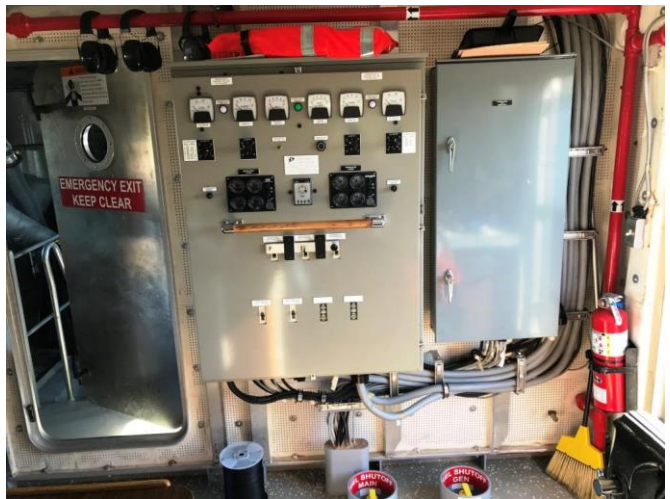
Photo # 22 – Main switchboard
