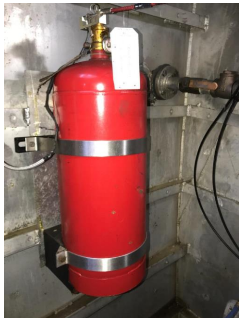
Photo # 54 – Comp. # 5 – Fixed fire system
