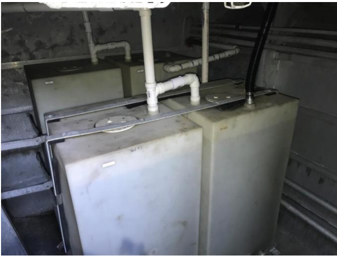
Photo # 55 – Comp. # 6P – 2 x 100-gallon sewage & 2 x 100 gallon fresh water tanks
