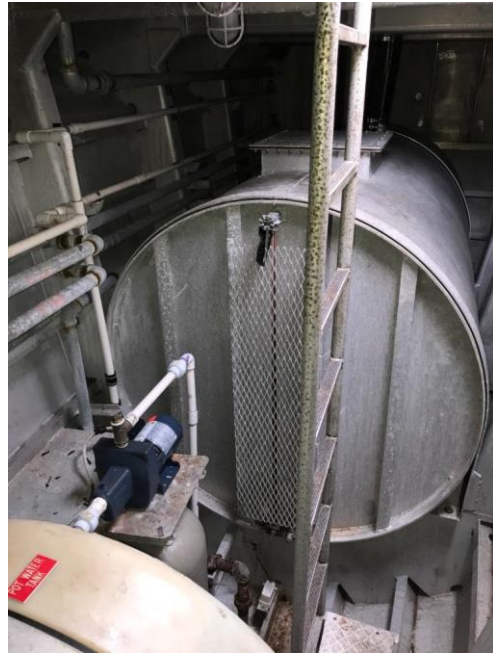
Photo # 44 – Comp. # 3 - Main fuel oil storage tank
