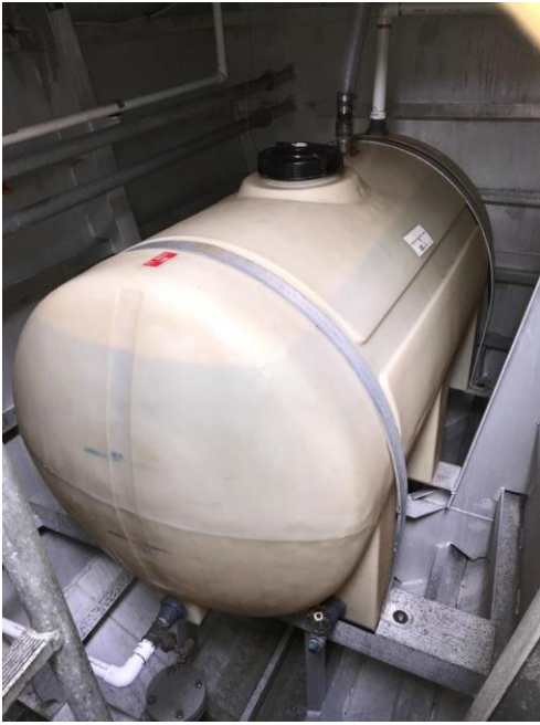
Photo # 43 – Comp. # 3 – 300-gallon fresh water tank
