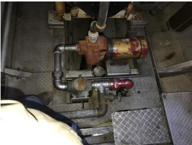
Photo # 53 – Comp. # 54 – 5.0 HP min fire pump
