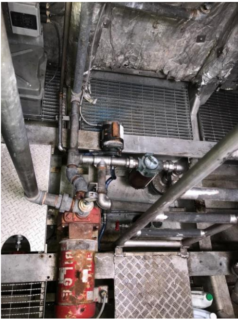
Photo # 51 – Comp. # 4 – 7.5 HP min fire pump
