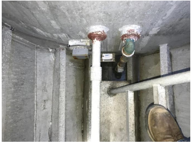
Photo # 44 – Comp. # 2 – Bilge suction piping and bilge alarm
