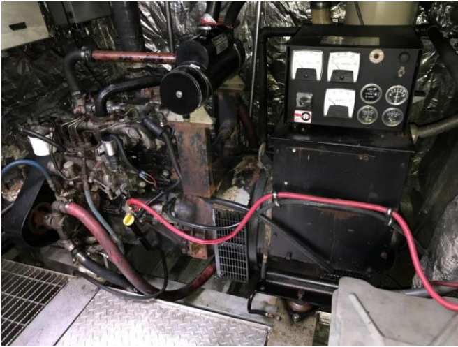
Photo # 47 – Comp. # 4 – 40 kW Generator Set
