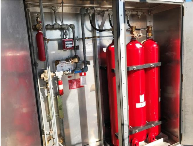
Photo # 19 – Fixed fire system on deck house roof
