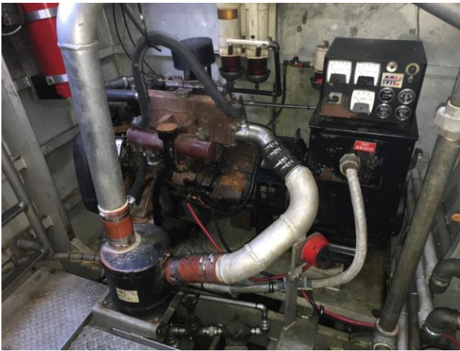
Photo # 49 – Comp. # 5 – 40 kW Generator Set
