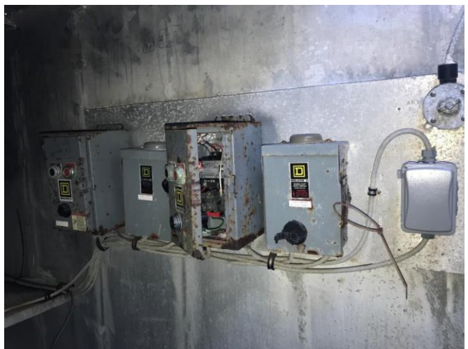
Photo # 60 – Comp. # 3P – Condition of various electrical starters, components, and exposed connections
