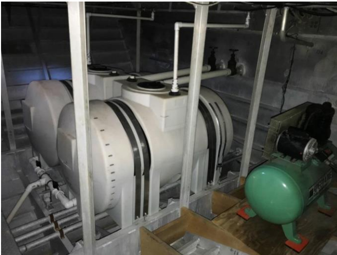
Photo # 39 – Comp. # 3 – Sewage tanks and air compressor
