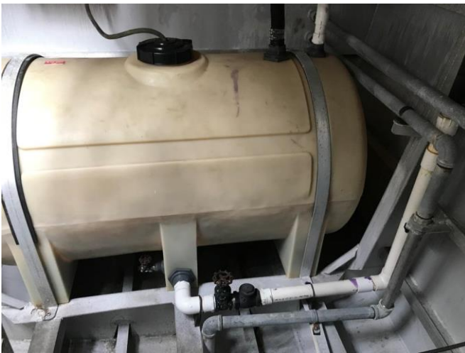
Photo # 53 – Comp. # 5 – 300-gallon sewage holding tank
